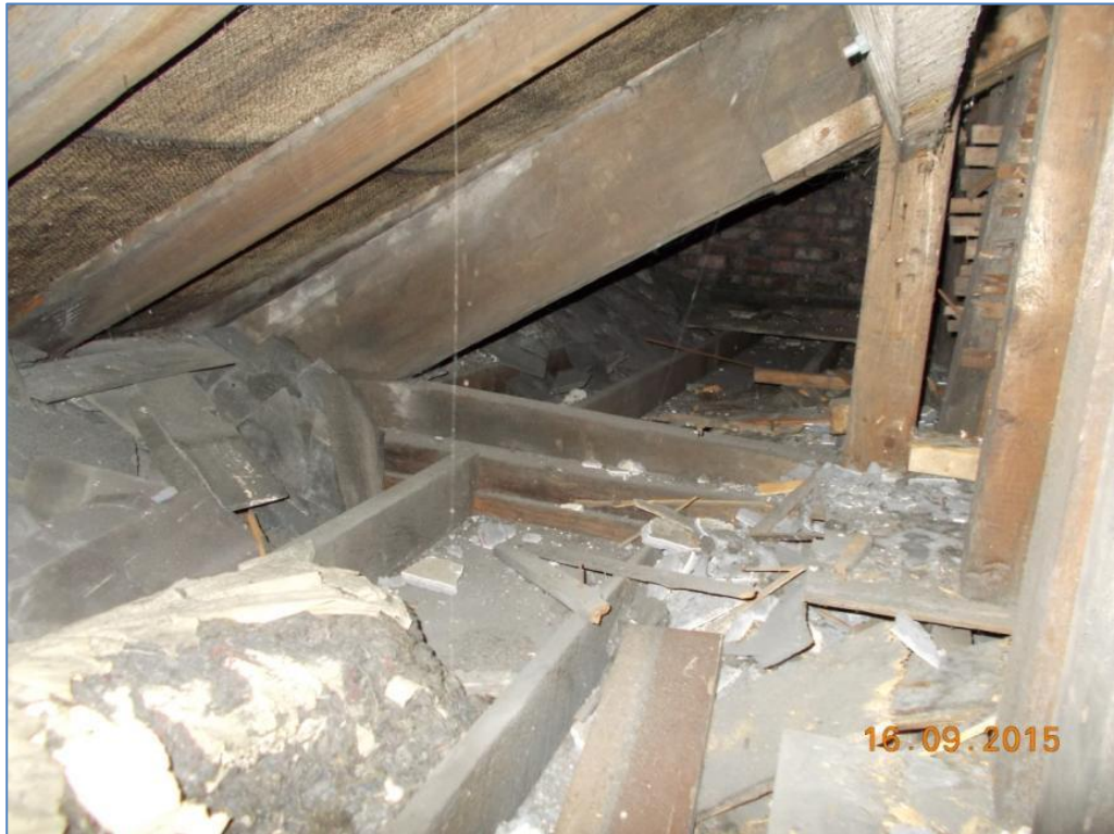
Photograph 4 - Low narrow roof void along eaves of main public house building.
