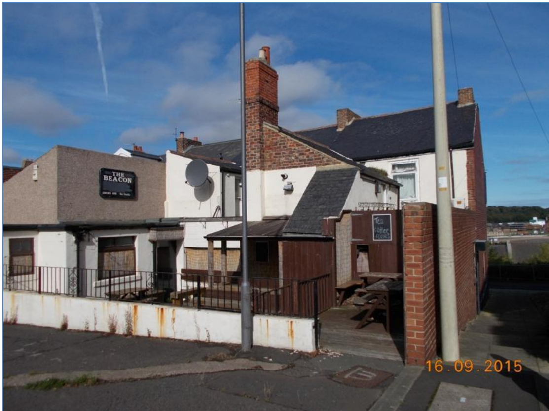
Photograph 2 – Rear (south) of the site.
