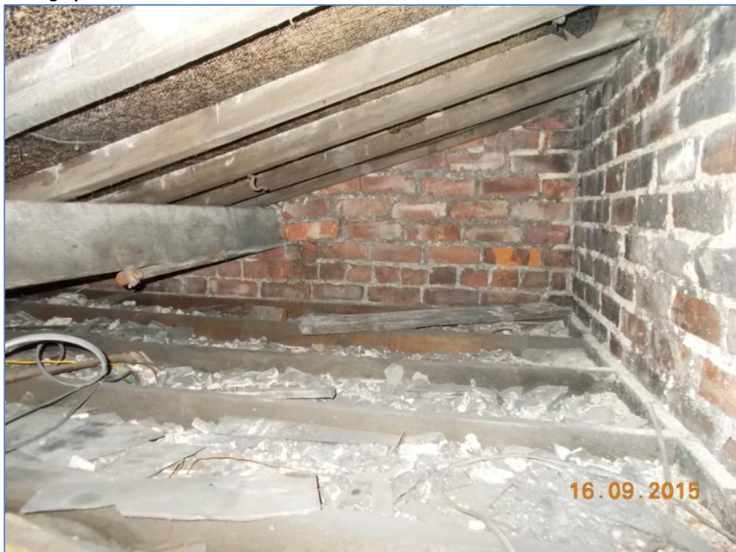
Photograph 6 - Roof void of extension to rear.
