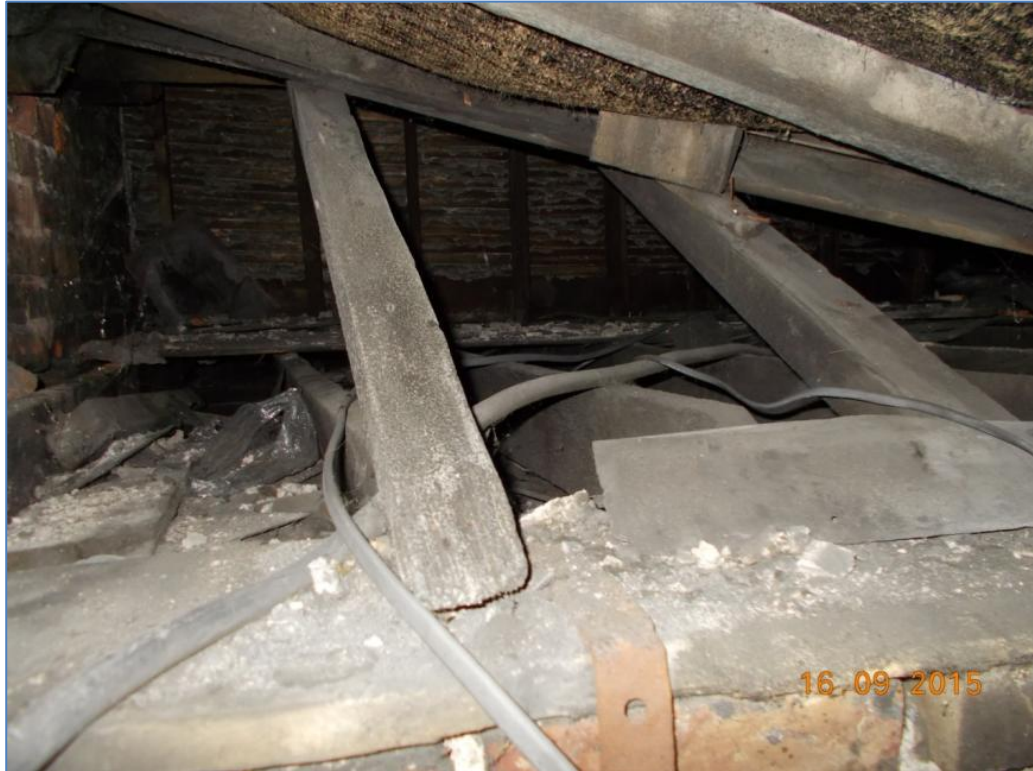
Photograph 5 - Roof void of extension to the rear.
